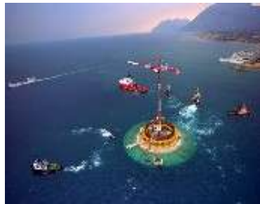
WET DOCK INSTALLATION M3 PYLON
